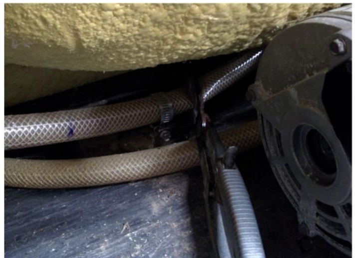
Jacuzzi J-350 with front cabinet removed. Circulation pump is behind the control box. Place one clamp between heater and flow switch. Place one clamp on suction line.
