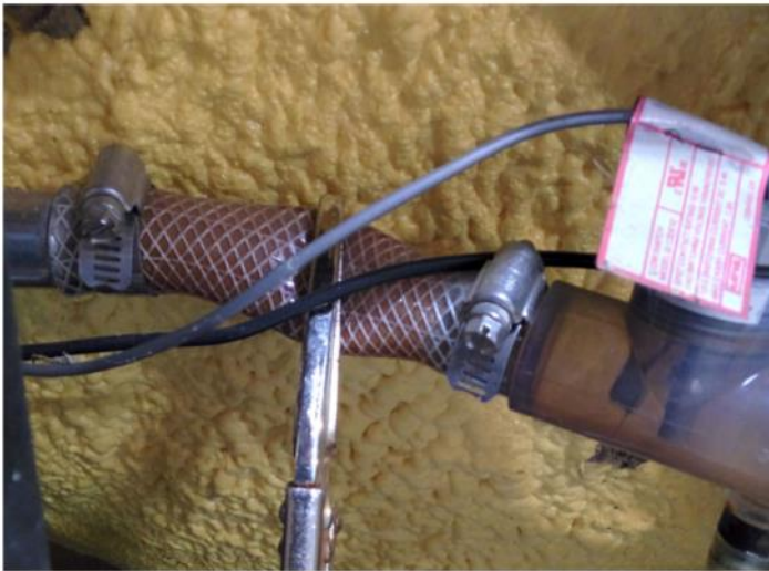
Jacuzzi J-350 with front cabinet removed. Circulation pump is behind the control box. Place one clamp between heater and flow switch. Place one clamp on suction line.
