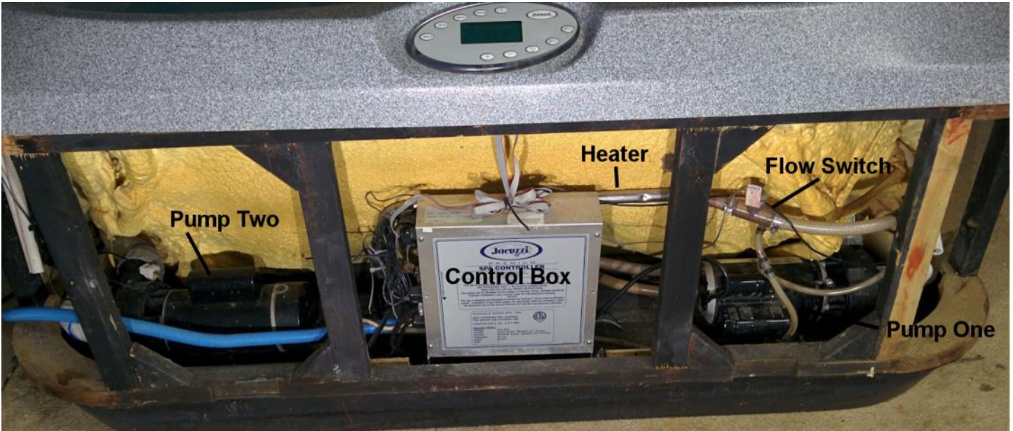
Jacuzzi J-350 with front cabinet removed. Circulation pump is behind the control box. Place one clamp between heater and flow switch. Place one clamp on suction line.
